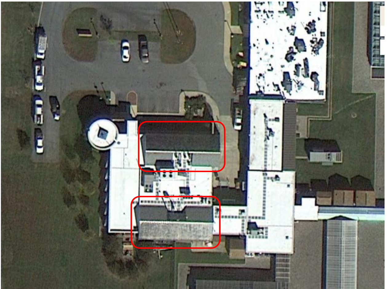
Figure 57: The two roofs of environmental concern at the APHIS complex
