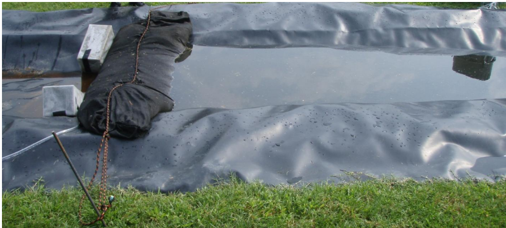
Figure 4: The Biommat placed across the swale, with influent stormwater visible on the right side
