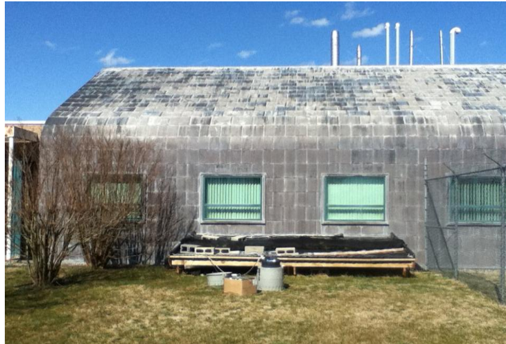
Figure 3: The roof runoff collection area
