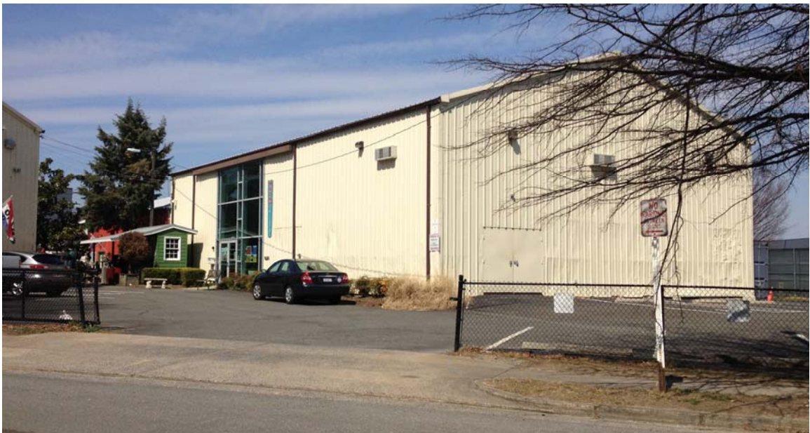
Figure 29: The MetroStage Theater is currently housed in a redesigned lumber warehouse at 1201 North Royale Street, immediately adjacent to the Tide Lock Park site. Photo by Erica Thum.
