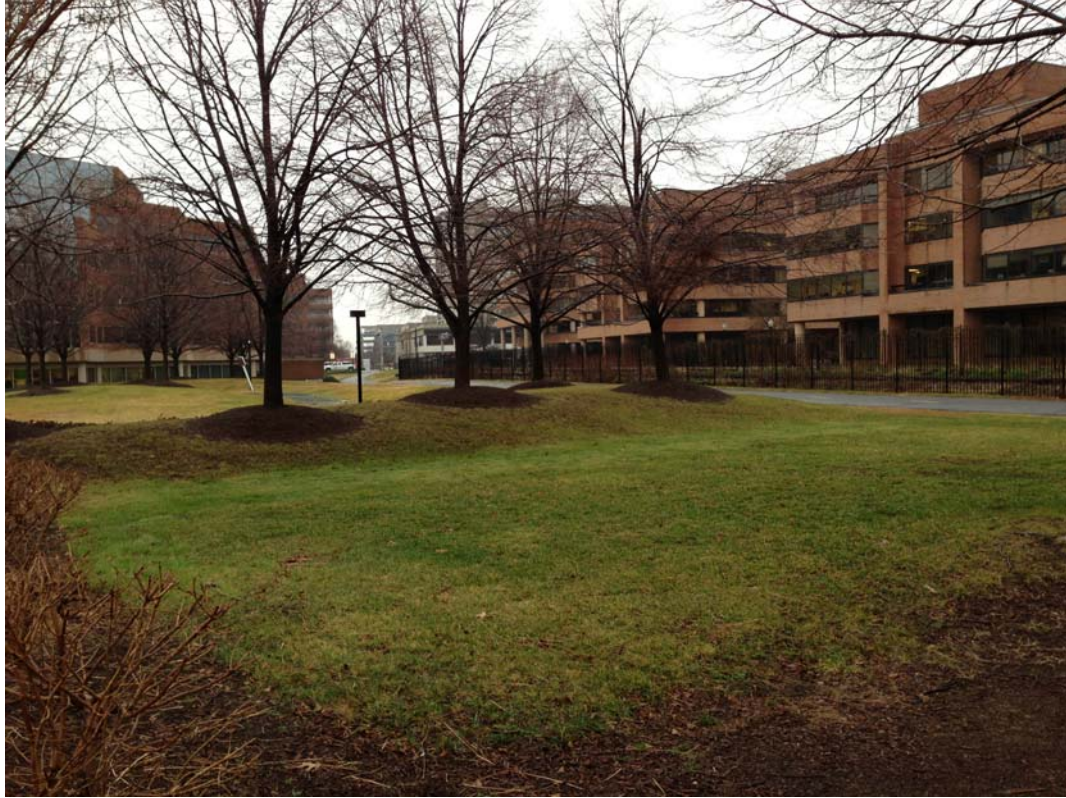
Figure 18: Photo of trees growing on mounds of earth on roof of underground parking garage. Photo by Erica Thum.
