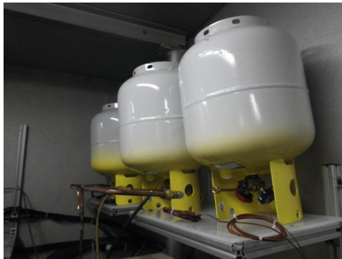
Figure 7: Expansion Tanks for Void Fraction Measurement
