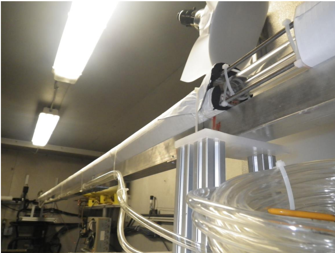
Figure 3: 1/4" Test Section Installed in System
