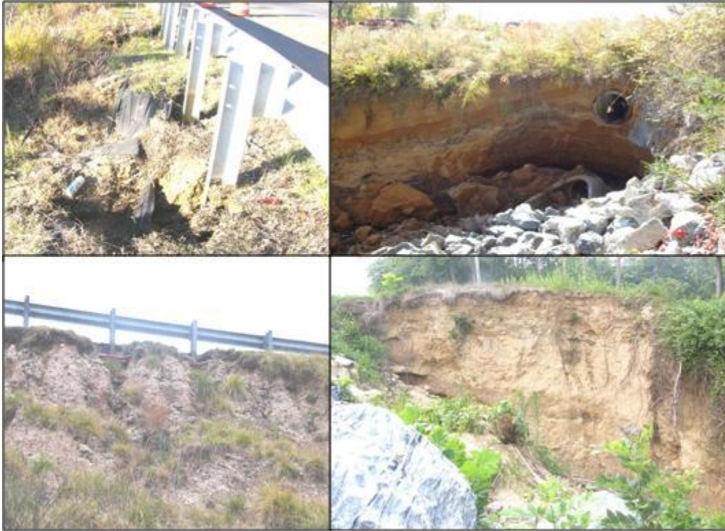
Figure 2.1: A collage of the different types of slope failures that have occurred in the State of Maryland
