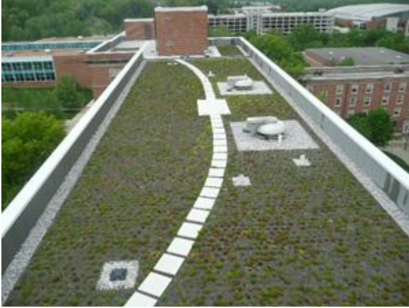
Figure 12: University of Maryland Cumberland Hall Green Roof
