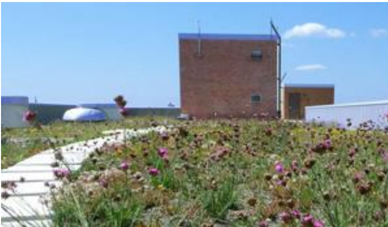
Figure 11: University of Maryland Cumberland Hall Green Roof
