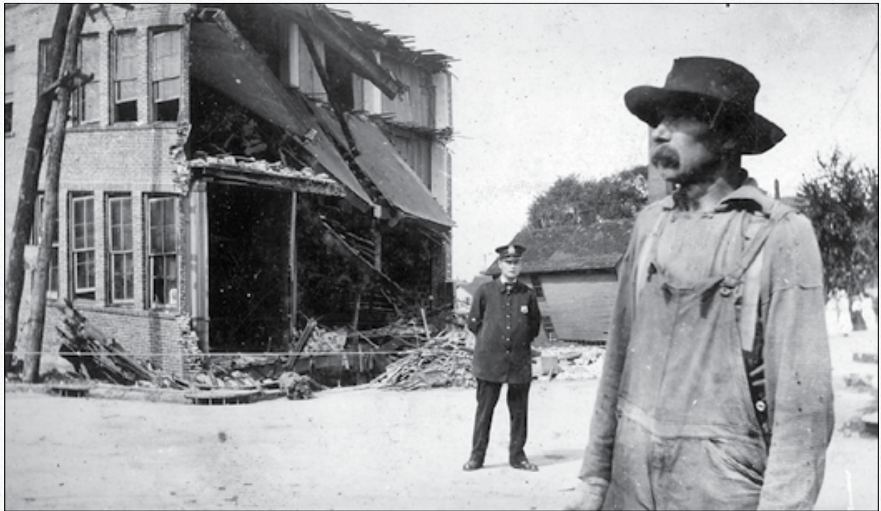
Surveying the damage after the Millcreek Flood of Aug. 3, 1915. Newman Photo Album, Erie County Historical Society.
