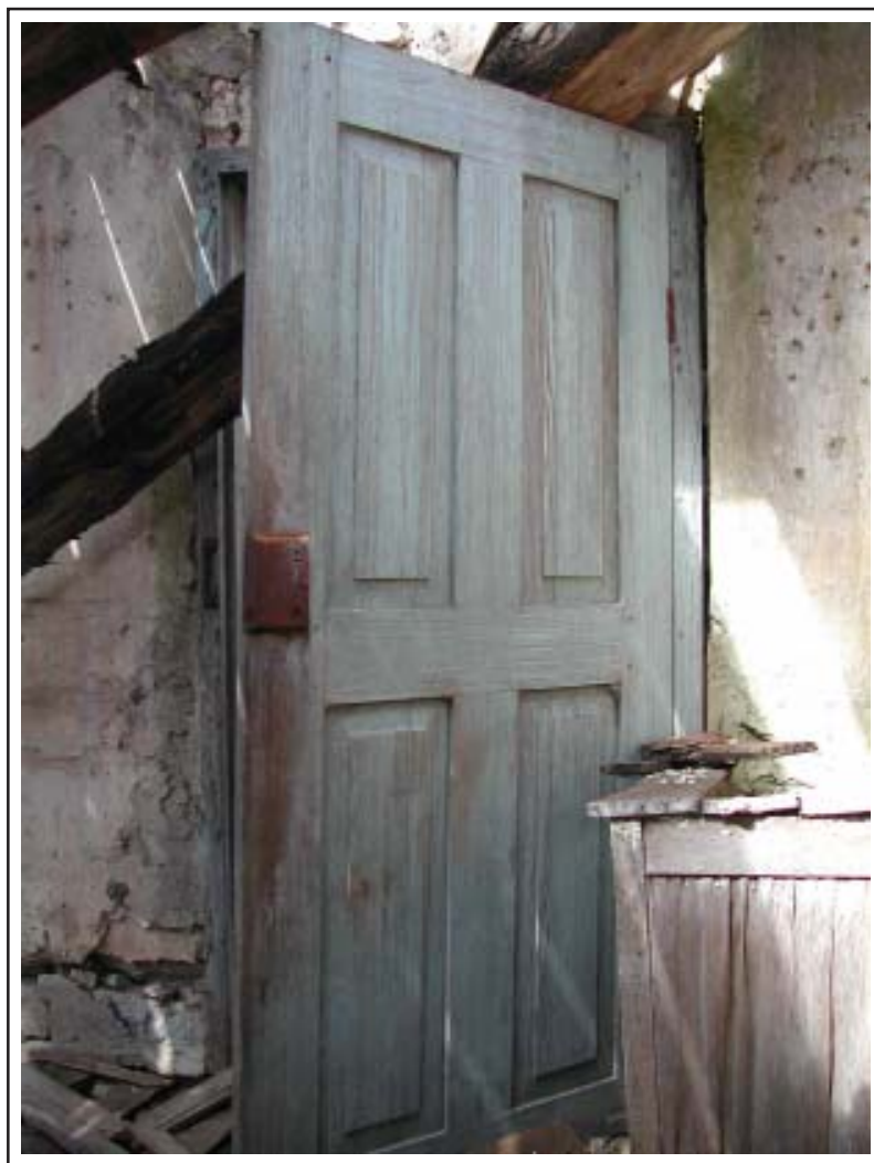
Figure 4.12. Light blue paint on interior door of the Jens and Kari Ringness House, Bosque County, Texas.
