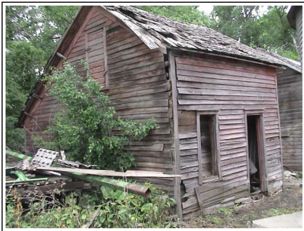
Figure 4.3. Front and west side facade, Goulson frame house, ca. 1880.
