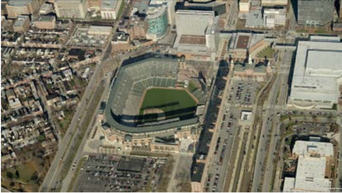
Fig. 6.1 – Oriole Park at Camden Yards, Baltimore, MD. aerial of stadium within its context. (2012) (Bing Maps)
