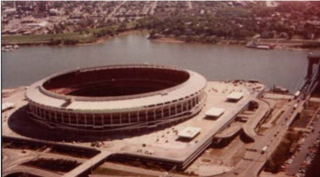
Fig. 2.3 - Riverfront Stadium, Cincinnati. aerial of tall, circular concrete form. (c1980) ( http://www.flickr.com/photos/brent_nashville/110006713/sizes/o/in/photostream/ )
