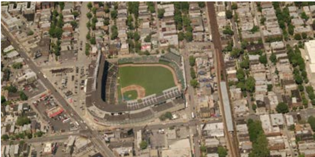
Fig. 2.2 - Wrigley Field, Chicago. aerial showing stadium conforms to street grid. (2012) (Bing Maps)
