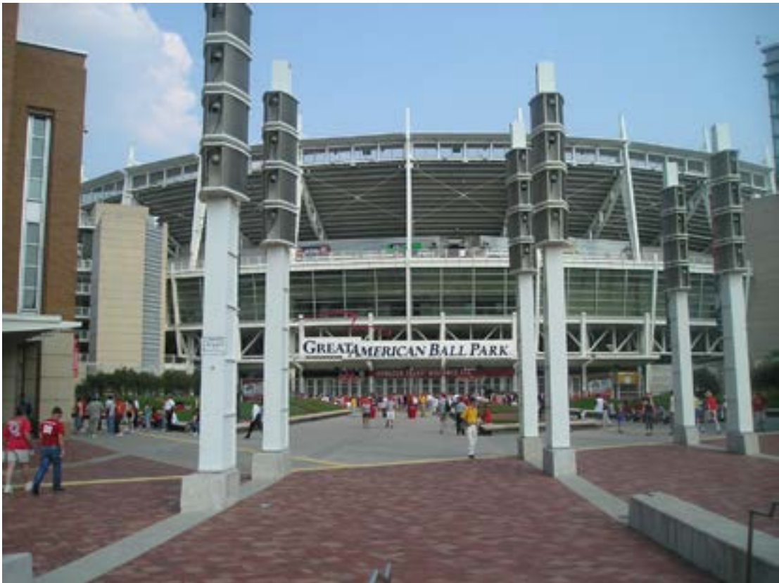
Fig. 2.7 – Great American Ballpark, Cincinnati. entrance showing glass façade. (2011) ( http://www.flickr.com/photos/39669102@N07/5726884987/ )
