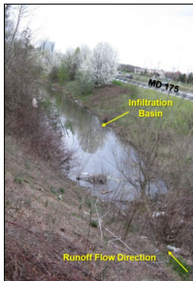
Figure 1. Photograph showing the infiltration basin located along MD 175 East. Photo, looking west, shows single concentrated inflow point to the infiltration basin.
