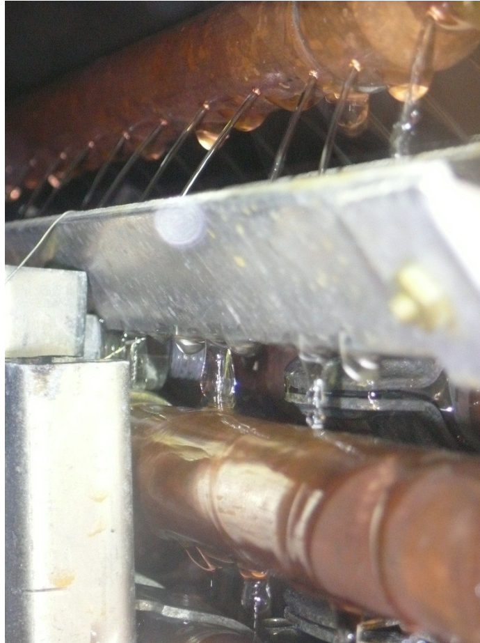
Figure 68: Falling film distributor in operation, close up
