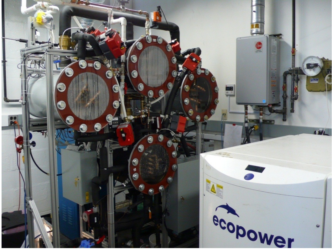
Figure 59: Prototype adsorption chiller near final configuration
