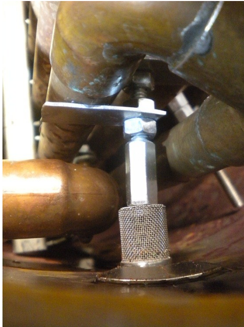
Figure 72: Inlet screen (230 micron) and magnet for refrigerant recirculation line
