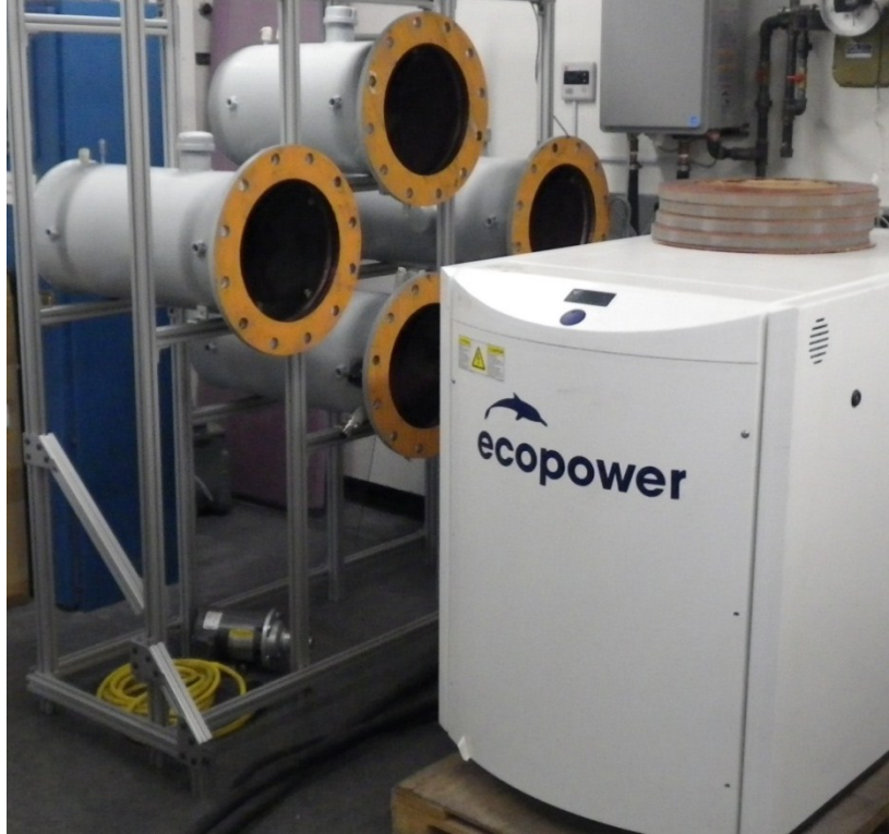
Figure 65: Vacuum chambers ready for heat exchanger installation, plumbing and instrumentation
