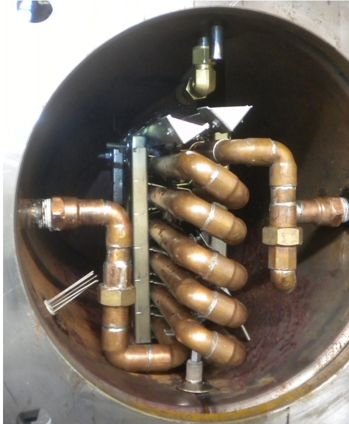
Figure 67: Falling film evaporator plumbed to chamber feedthroughs
