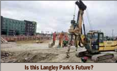
Is this Langley Park's Future?
