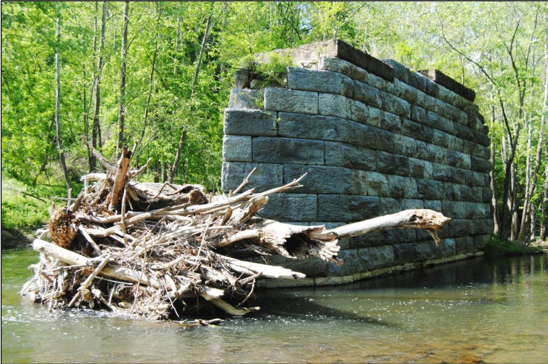
**Figure 27. Stone bridge abutments from an earlier B&O Railroad alignment (Photograph by Sarah Pickard).**
