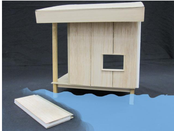
Figure 59 Elevating the building on concrete piles will protect it against small floods.
