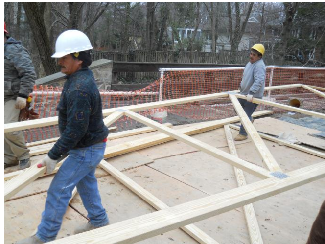
Figure 55 Components should be constructed to easily be handled with only man-power.
