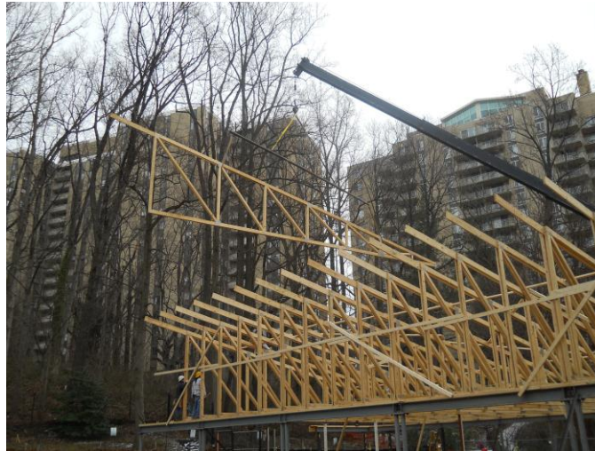
Figure 54 Large machines cannot be counted on for construction.
