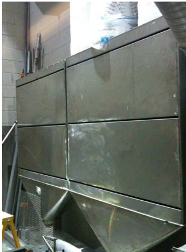
Figure 2-2. Ventilator for sodium fumes
