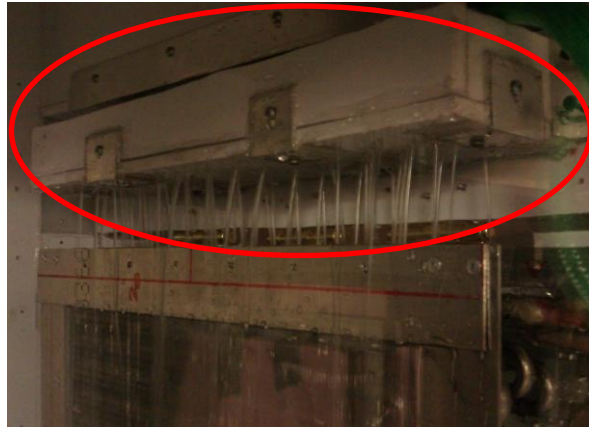
Figure 33: Wetting Water Distributor
