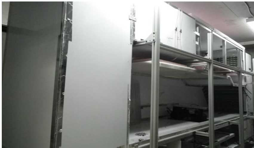
Figure 22: The Existing Air Duct in CEEE Lab.
