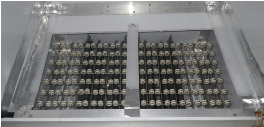
Figure 42: Electrical Air Heaters
