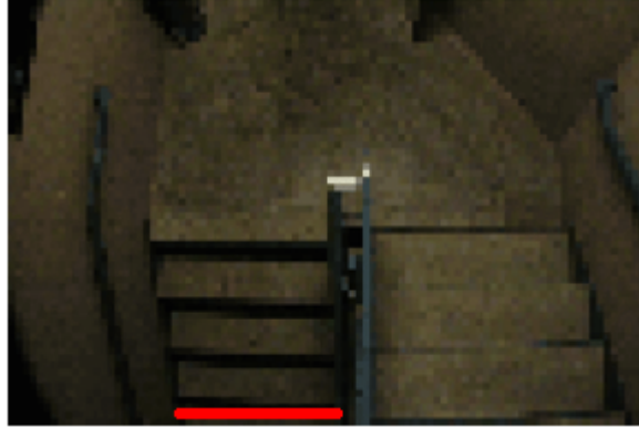
Figure 4-1: Exit Point in Stairs in Building 4
