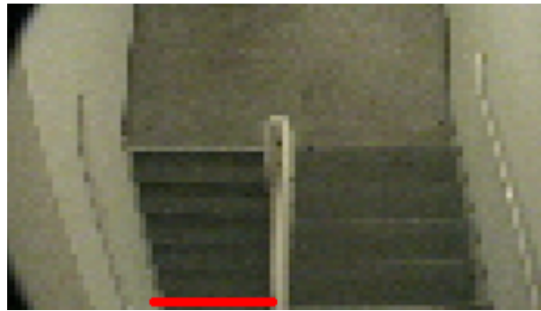
Figure 4-2: Exit Point in Stairs in Building 5
