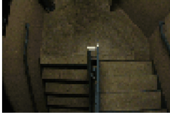
Figure 3-1: Building 4 Typical Camera View [34]
