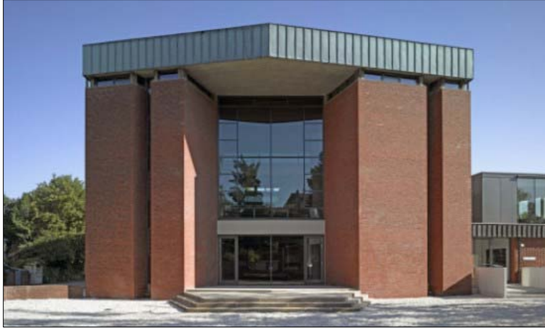
Figure 37: Exterior view of St. Bonifatius after the adaptive reuse, note the clear glass (Christian Richters, http://www.agn.de/popup.php?pid=602 )
