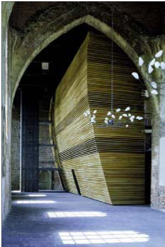
Figure 4: Interior view of Sankt Marien towards the addition (Courtesy of Klaus Block Architekt, www.klausblock.de )
