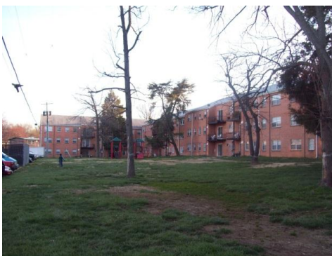
Figure 16 A Courtyard Surrounded by Garden Style Apartment, author
