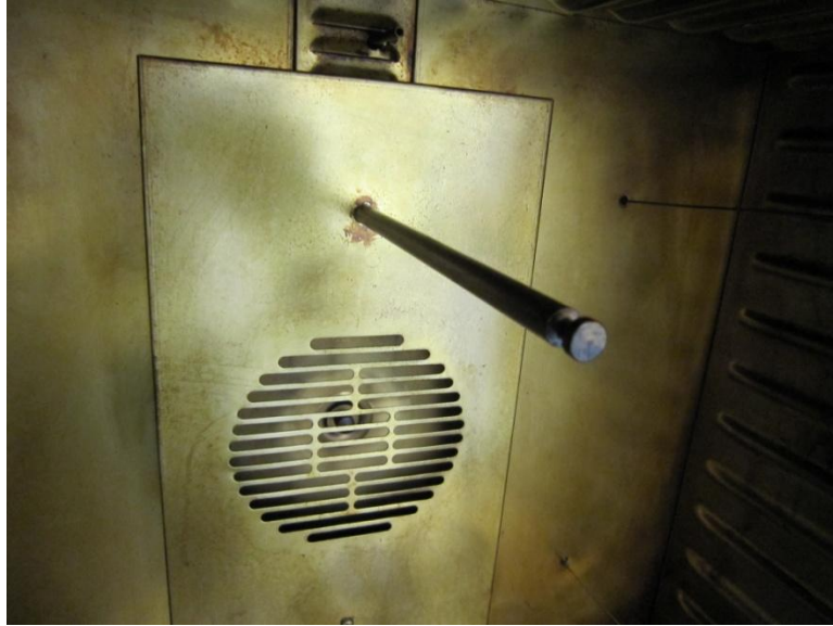
Figure 3.4: Hanging Rod Installed Above Fan in Oven
