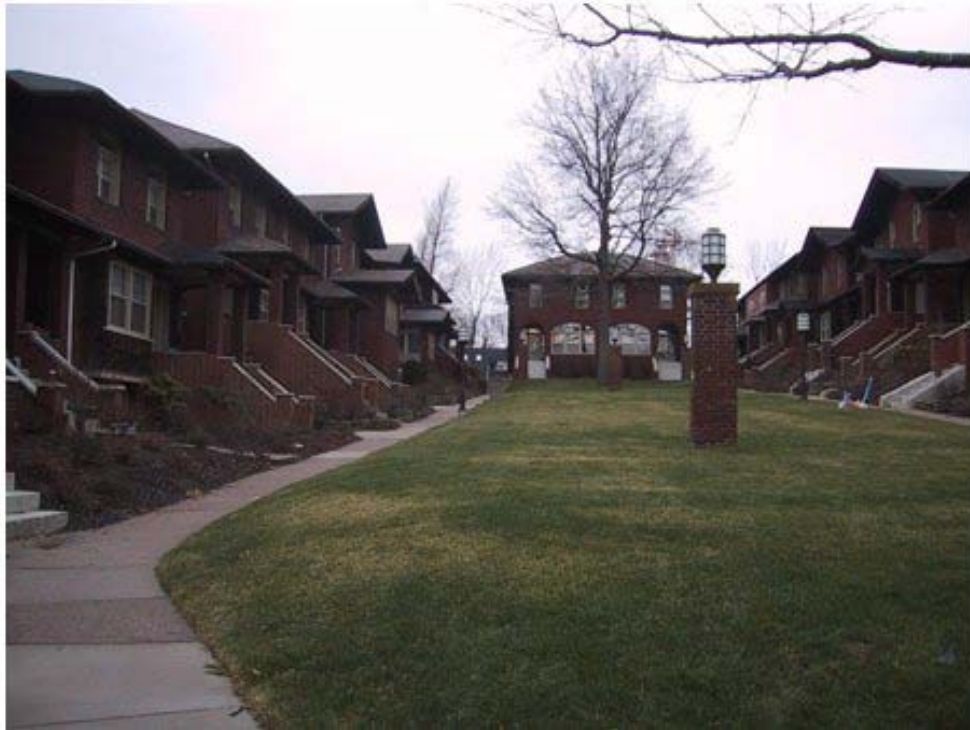
Fig. 31. Forbes Terrace after tree removal (photograph by Sharyn Frederick)
