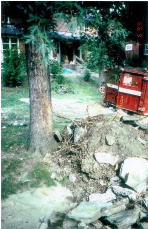
Fig 60. The razing of Beacon Gardens central courtyard to make room for a parking lot (photographer Sharyn Frederick)
