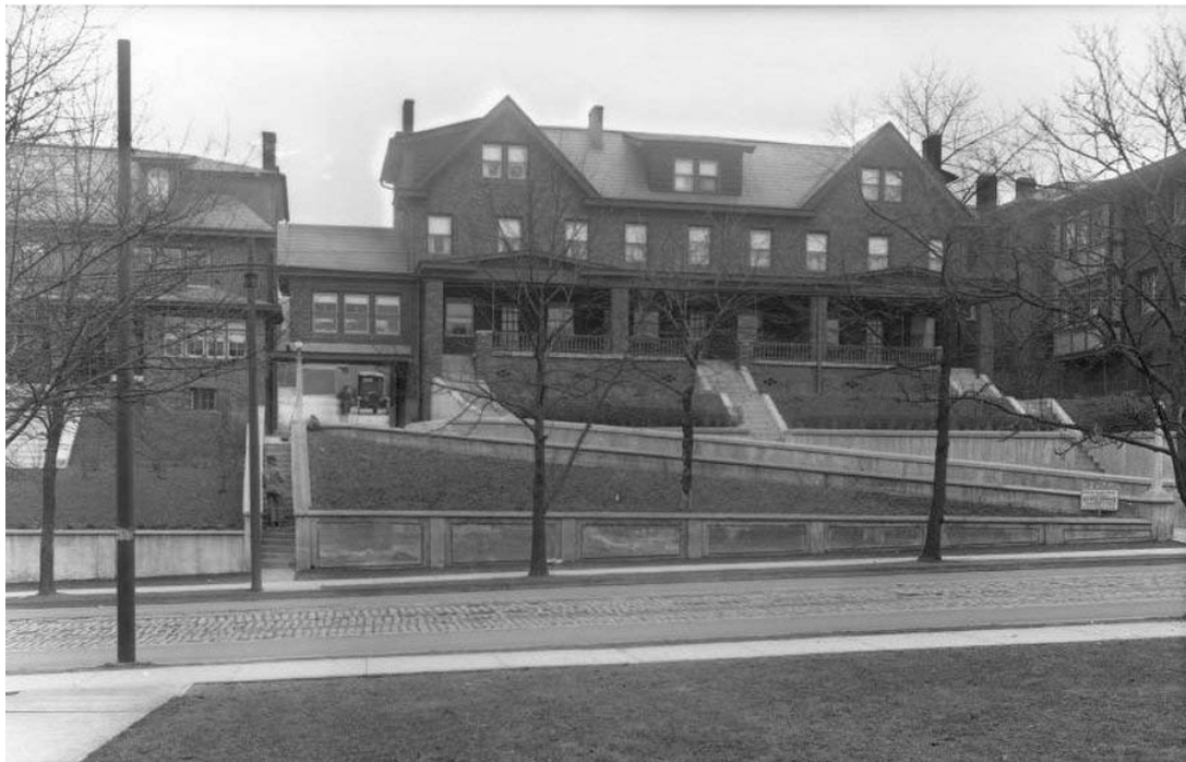
Fig. 8. Forbes Terrace, circa 1921 (courtesy of the Pittsburgh City Photography Archives). This view omits the courtyard entrance, which is to the right. An automobile is captured ascending to the parking garages that were integrated into the original site design.
