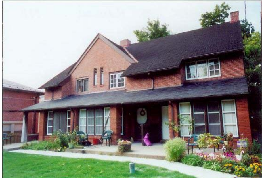
Fig. 26. Dan's house that retains nearly all of the original features of Scheibler's plan (photograph by author)
