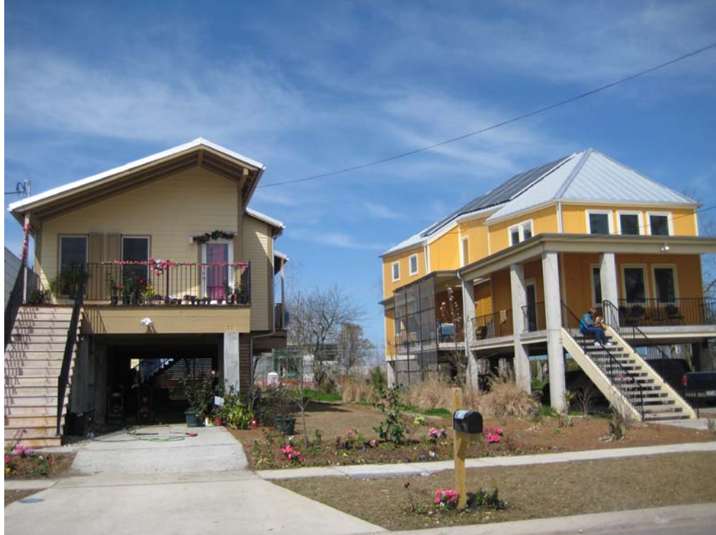
Figure 10 Image of Make it Right houses, author
