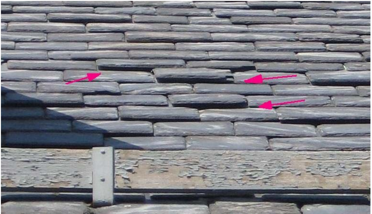
Fig 21 Photo showing results of nailing tops of slates too tightly. Photograph by author.
