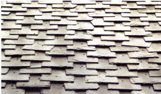
"Open Slating" shown on a Spanish roof (above)
