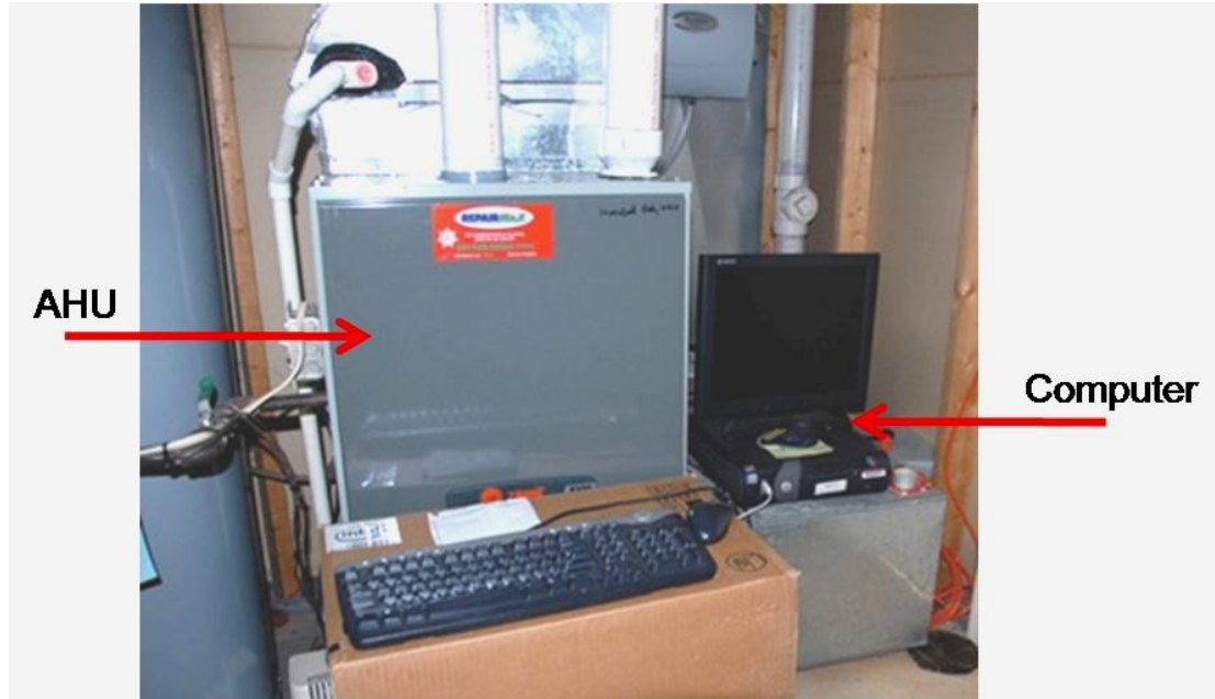
Figure 3.13 Photograph of the AHU and Control System Computer
