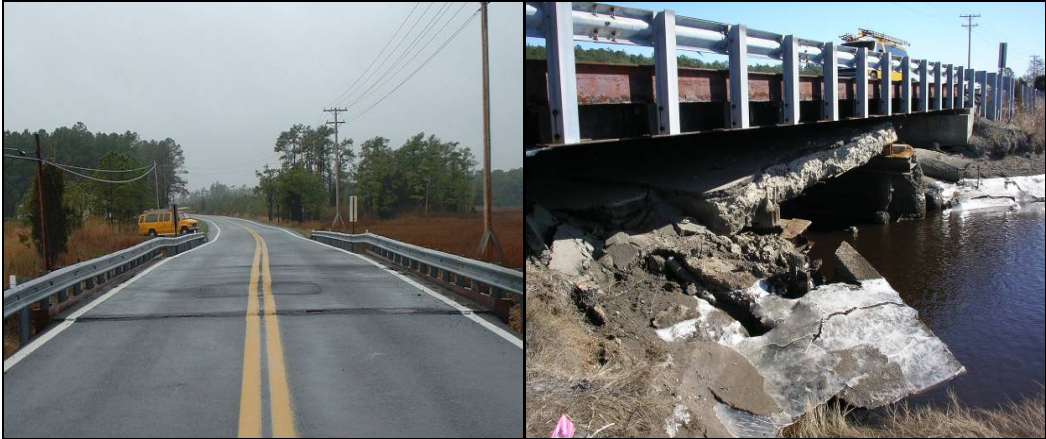
Figure 1 - Structure No. 0901100 Wallace Creek Bridge (Old)
