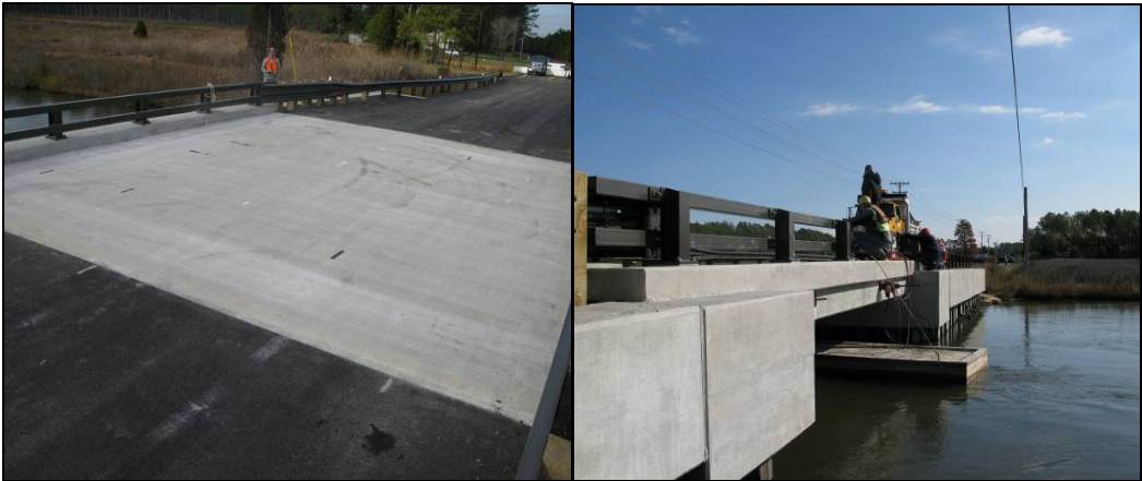
Figure 2 - Structure No. 0901100 Wallace Creek Bridge (New)
