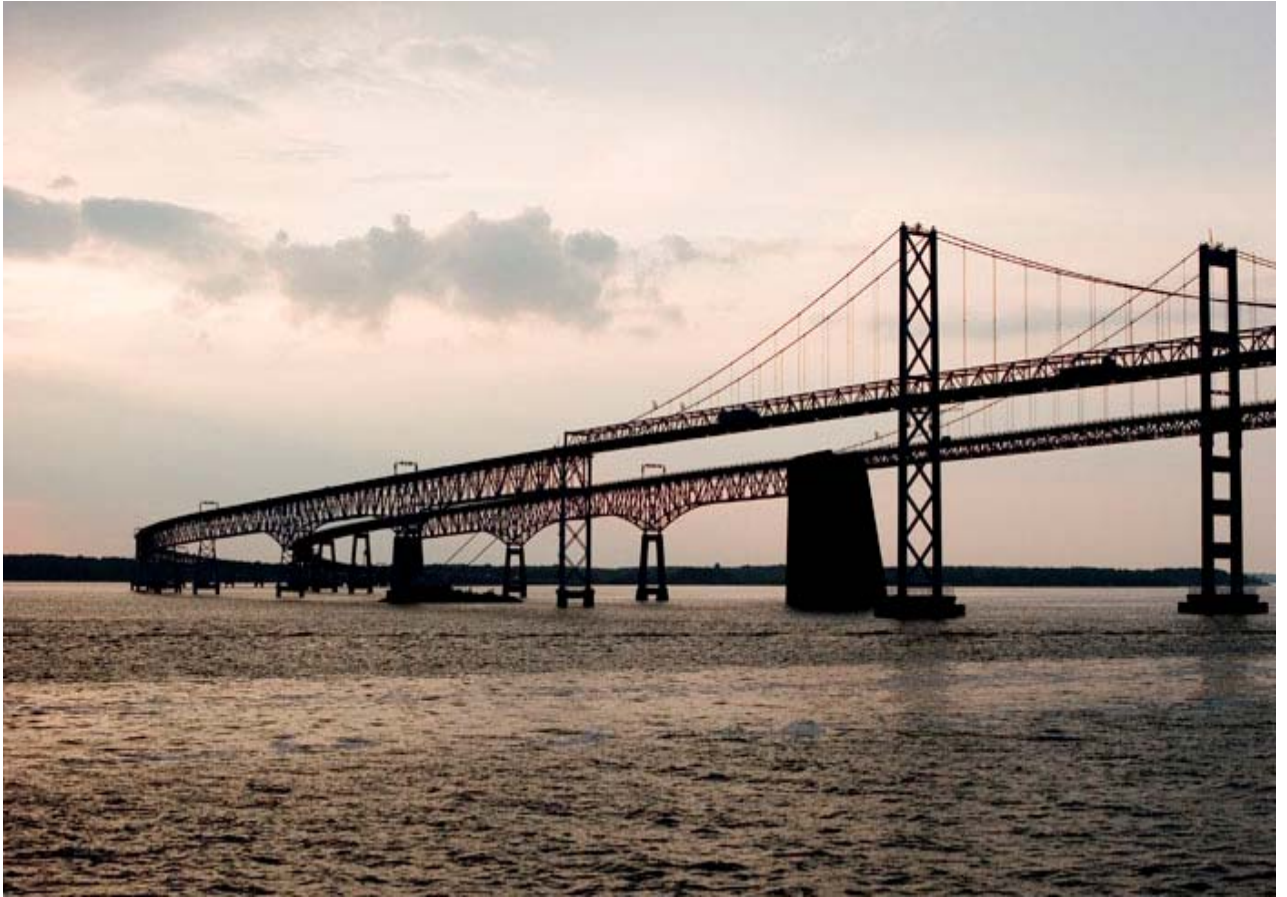
Figure 1.1. William Preston Lane, Jr. Memorial Bridge
