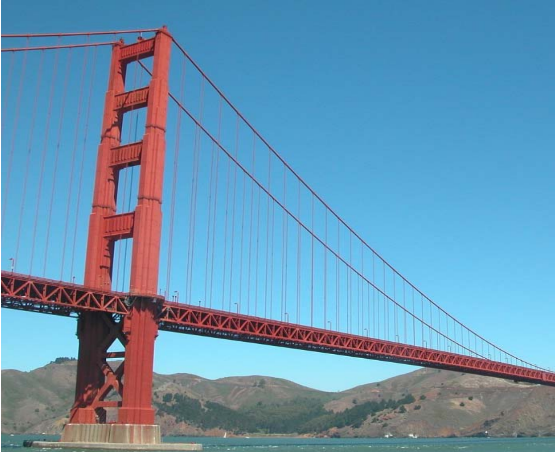
Figure 2.2 Tower of suspension bridge (Golden Gate Bridge, SF)
