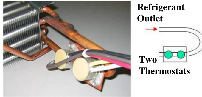
Figure 17: Defrost Control Setup
