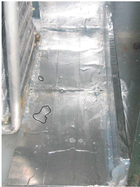
Figure 5.23 Drain Pan 90 Minutes into an Off-cycle
