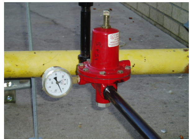
(b) Regulator#2 before the compressor set at 10 psig
