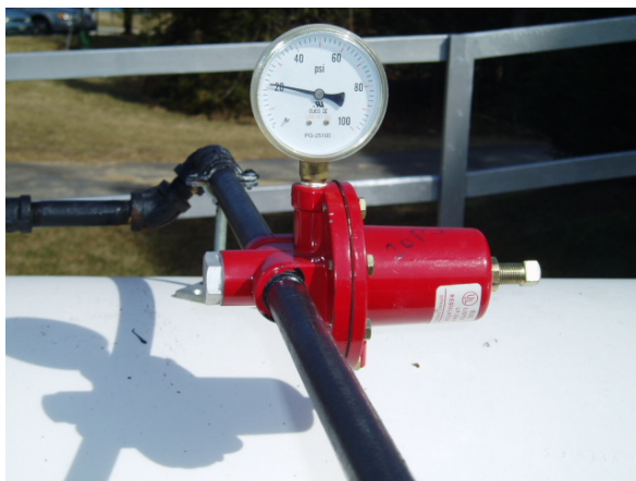
(a) Regulator#1 right after the propane tank set at 22~25 psig
