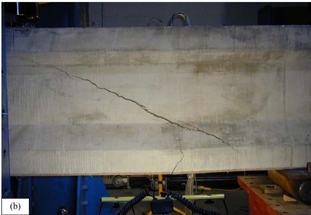
Figure 6.2.3-I: Girder 14S at (a) peak load and (b) post-peak load of 595 kips
