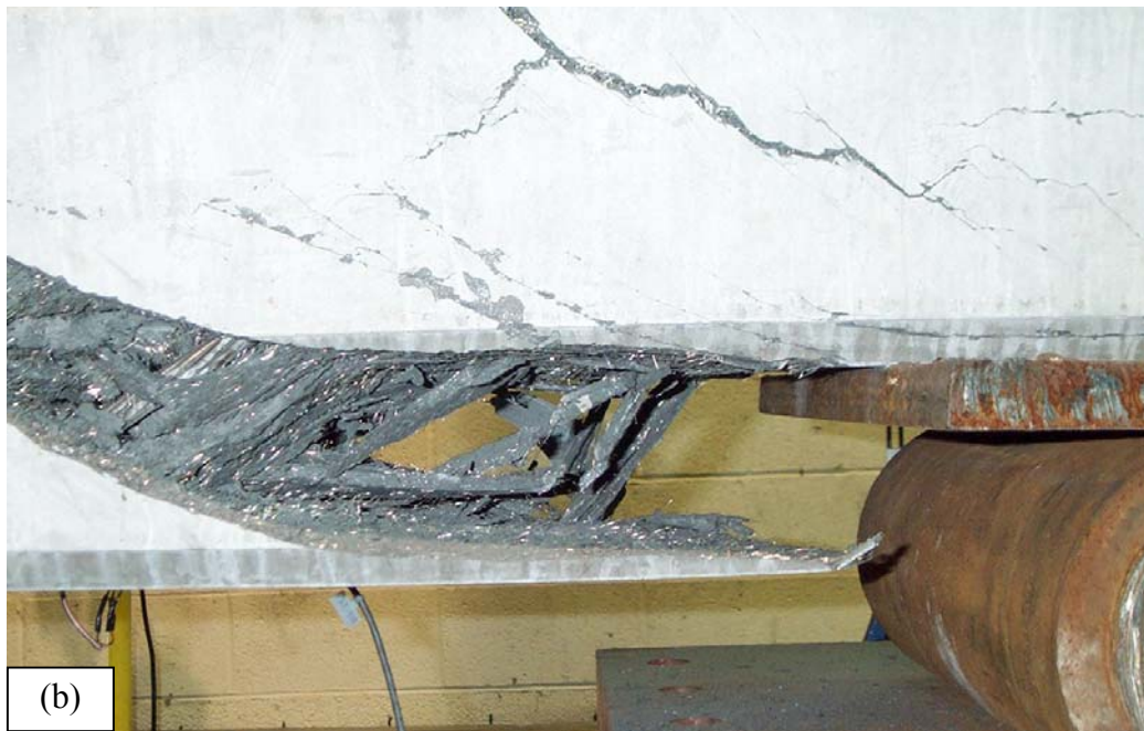
Figure 6.2.2-I: Failed Girder 24S (a) south elevation and (b) bottom flange near bearing
