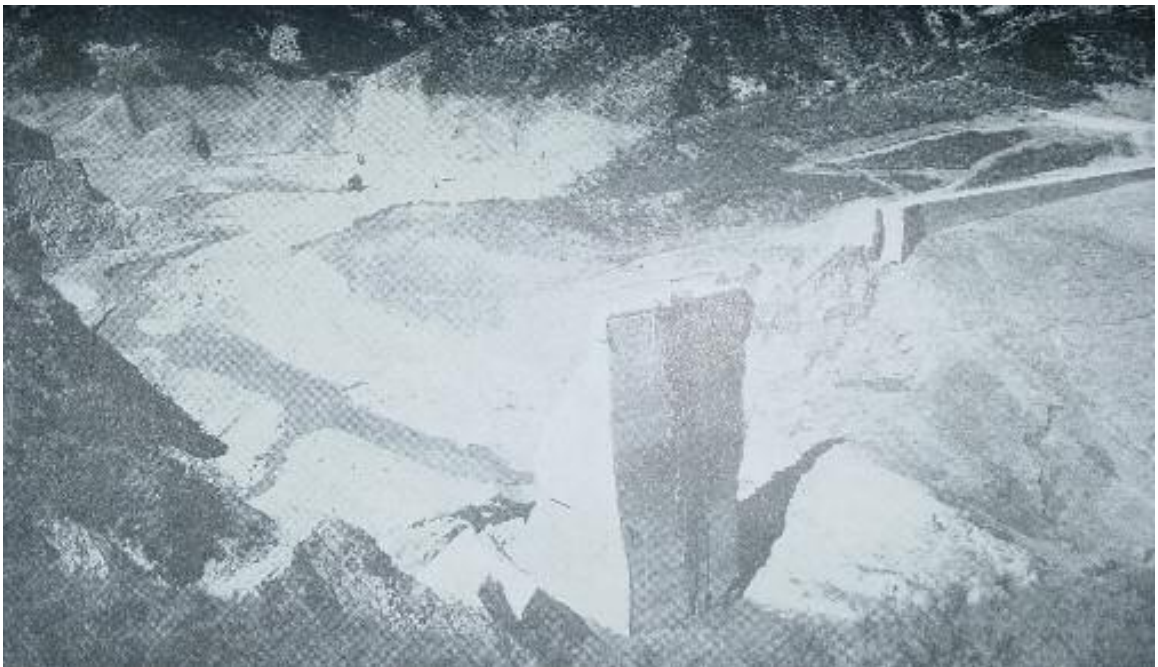
Plate 17 View from upstream side of St. Francis Dam after collapse.
