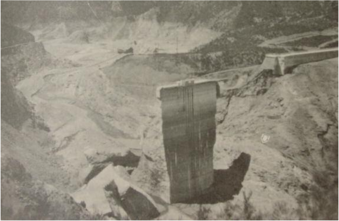
Plate 1 Fault line visible in picture taken after the St. Francis Dam collapse.
