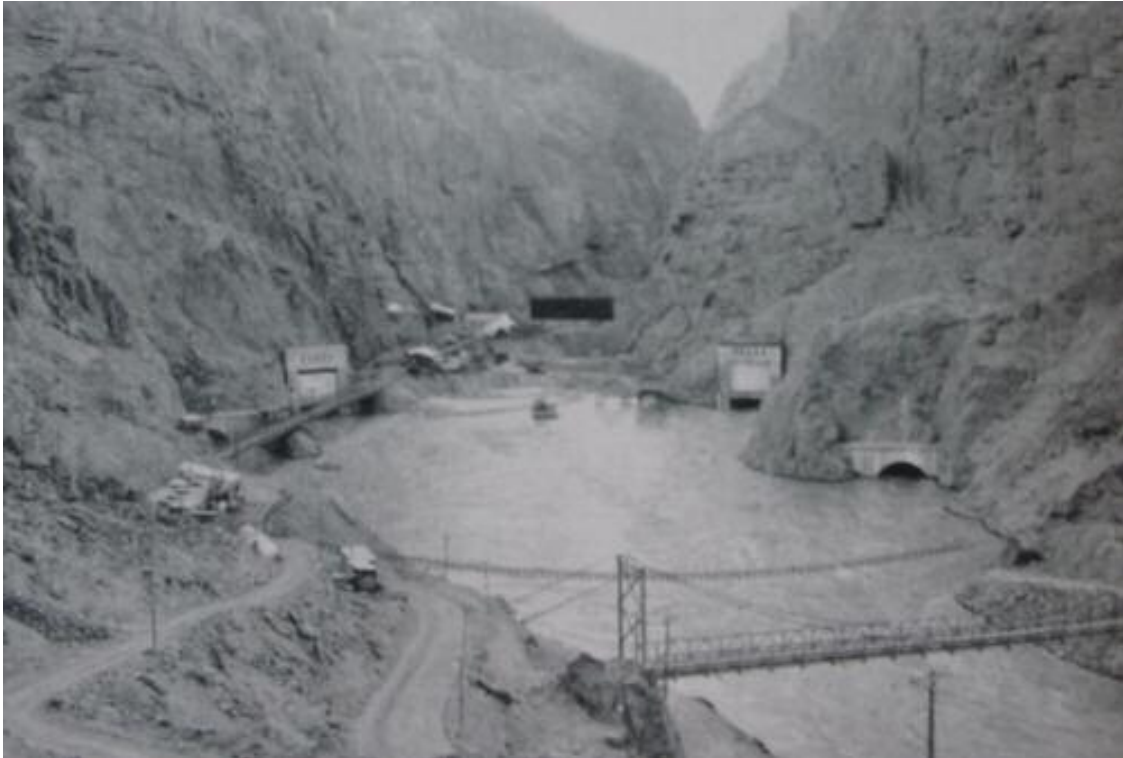
Plate 14 Three hundred foot long cooling plant (black building) located on lower coffer dam.
