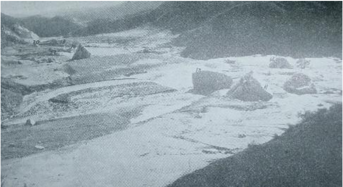
Plate 2 Location of St. Francis Dam fragments after the collapse.
