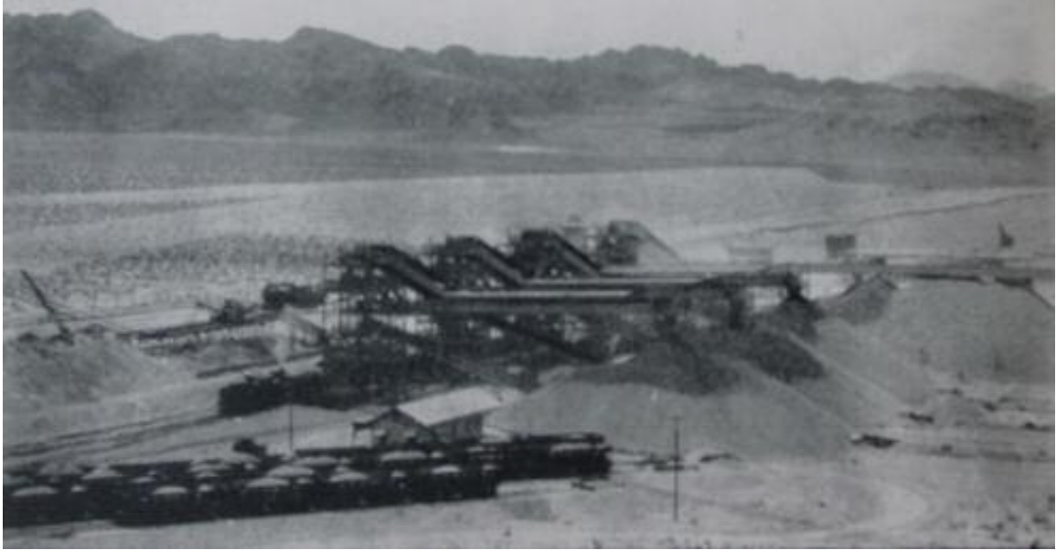
Plate 20 Hoover Dam sand and gravel screening plant.
