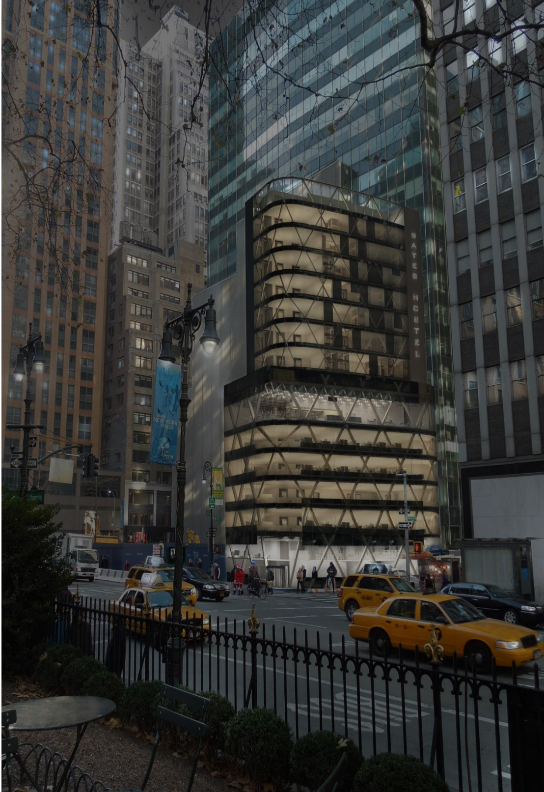
FIG 53: View of the Bates Hostel from Bryant Park Source: Author
