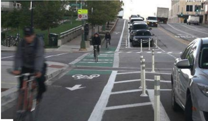
Figure 10 Buffered Cycle Lane on Busy Arterial in Chicago, Illinois. Source: http://spokesdunedin.wordpress.com/2012/11/10/protected-bike-lanes/ Accessed: May 05, 2013.
