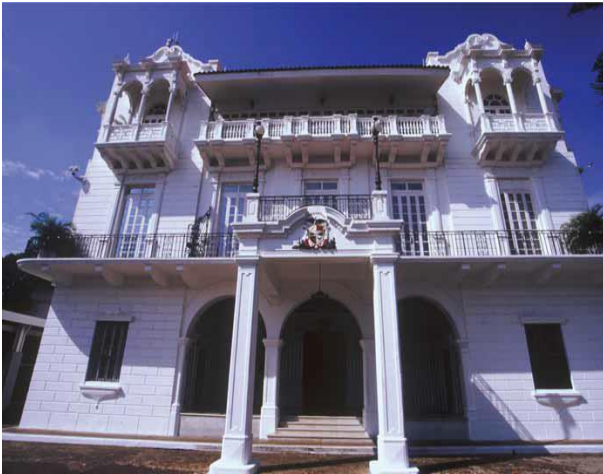
Figure 31 Example of Institutional Building Source: Vanessa Spadafora
