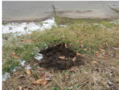
Source: Author Fig. 54. Buried Grate
