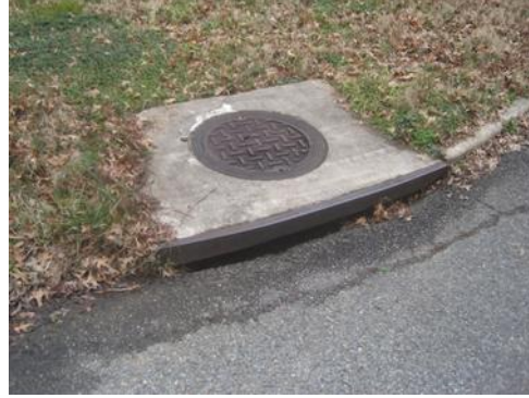
Source: Author Fig. 52. Existing Sewer Inlet
