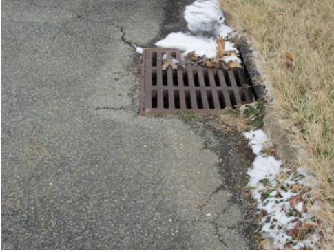
Source: Author Fig. 51. Existing Sewer Grate
