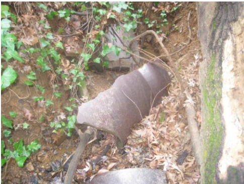
Source: Author Fig. 53. Damaged outfall
