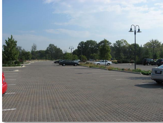
Fig. 20. Morton Arboretum Permeable Paver Parking Lot
