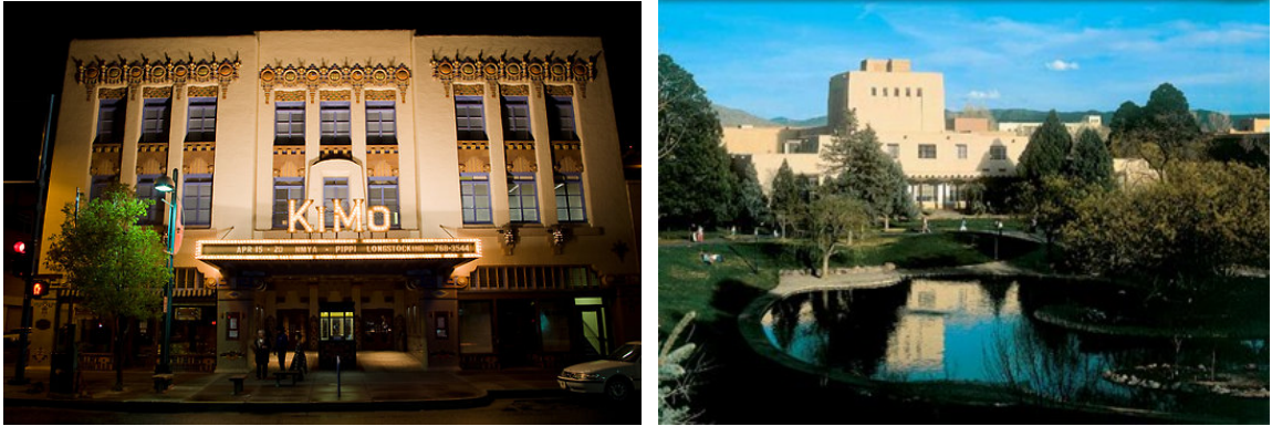
Figure 14 Kimo Theatre front façade (left) and Zimmerman Library original entrance facade (right) 24
