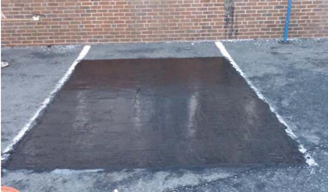
Figure 16. The completed sealant on the parking space before drying.
