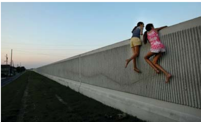
Fig.6_10: seawall @ New Orleans
